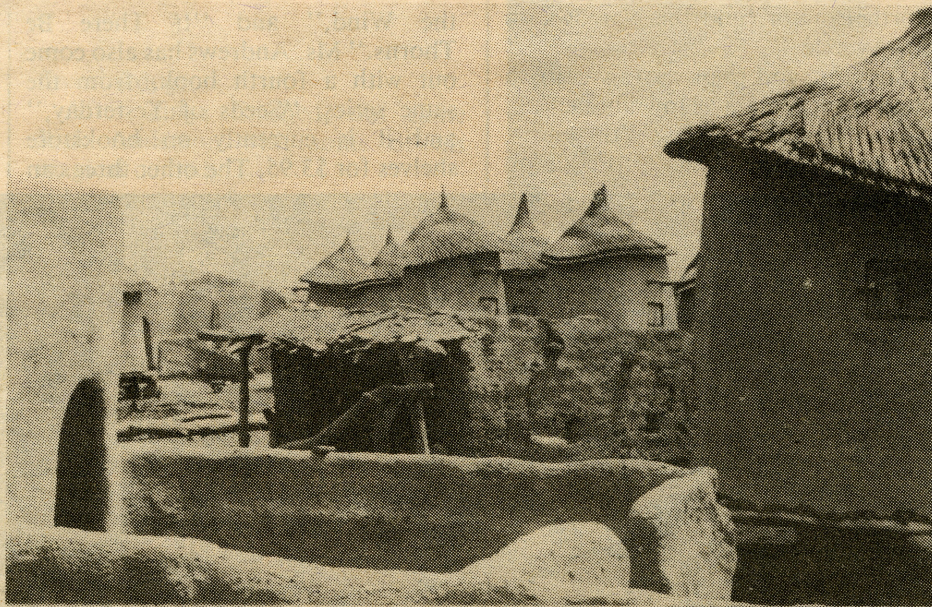
Silo rooftops in the upper Voltan village of Tialgo. Earthen walls up to 12 inches thick keep the houses cool inside.
