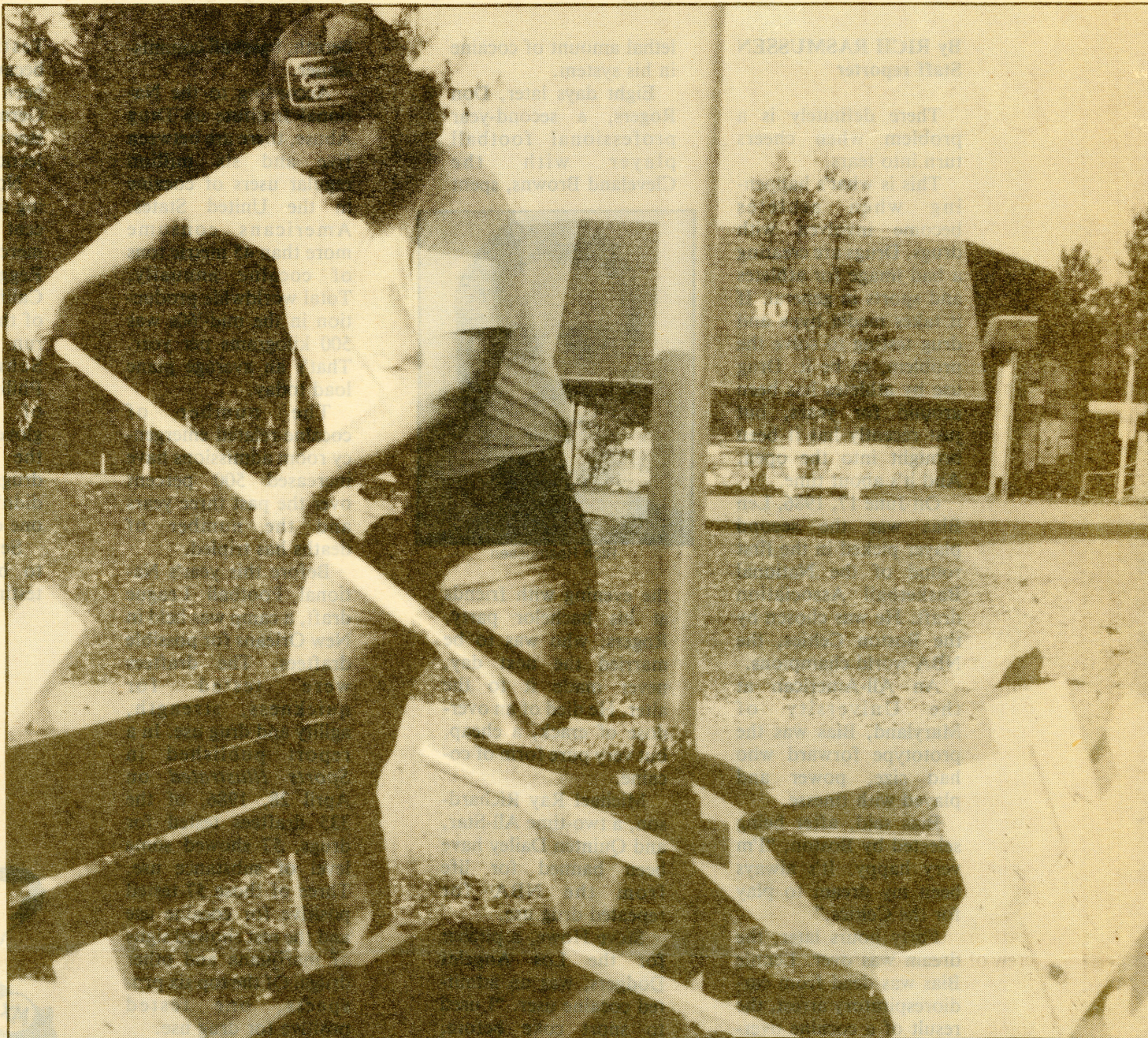
During infrequent breaks of good weather, there always is revamping to be done. At right, Mike Gillen, a maintenance department carpenter, temporarily switches trades to pour cement that will stabilize the foundation of one of the new benches that recently have appeared on campus.
