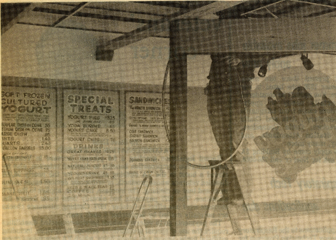
Putting in the light fixtures at 'the yogurt stand'.
