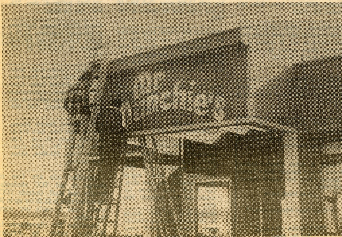
Workmen put up sign as a James Center restaurant nears completion.
