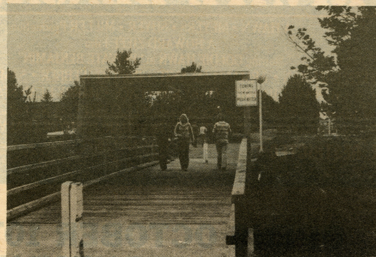
The new bridge
