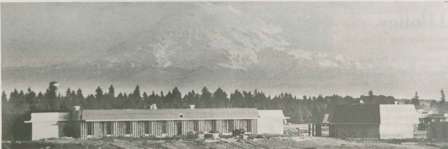
NEW BUILDINGS — Mount Rainier emerges from its cloud camouflage to be photographed as backdrop for new campus buildings. Seven buildings are now in use, and construction progress continues
